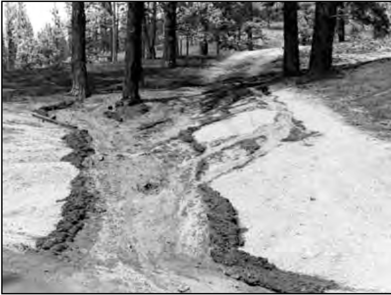
Soil erosion following fire photo U.S.F.S./B.L.M.
